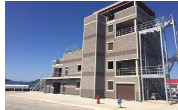
Fire Training Complex - Training Tower
